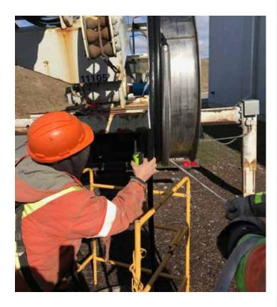
For the field trial, the same crew pulled two 3,456-fiber EDGE Rapid Connect Indoor/Outdoor Transport Trunks through the same type of 4-in duct along the same cable route. Lightwave's techs removed the reduced-diameter pulling grips on each end and revealed a new innovation from Corning and US Conec: 24-fiber Fast-Track MTP° Connectors, a staggering 144 of them in each 2-in grip.
